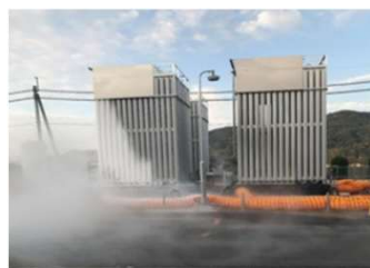
LNG vaporizer air-heating type conversion and reuse of cold heat
