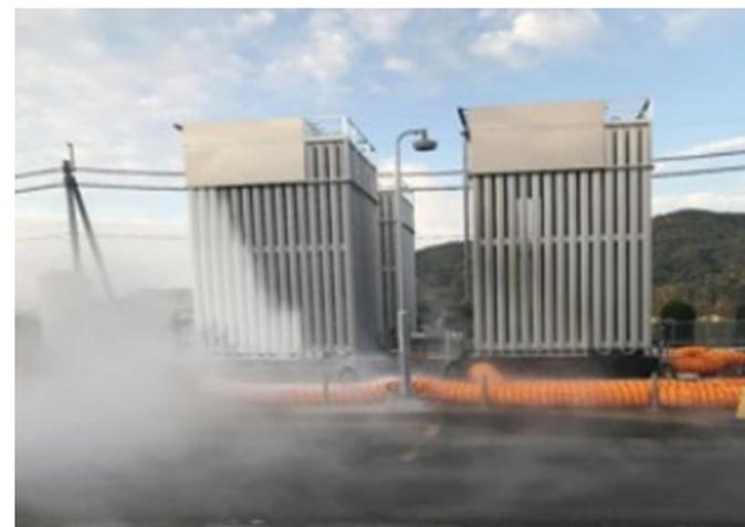
LNG vaporizer air-heating type conversion and
