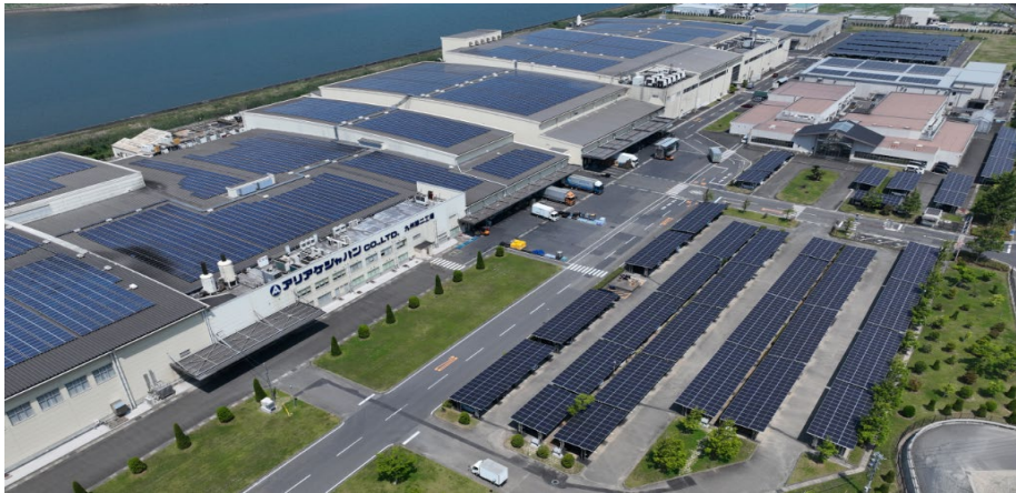
No. 2 Kyushu plant, Self-consumption type solar photoelectric generation system
