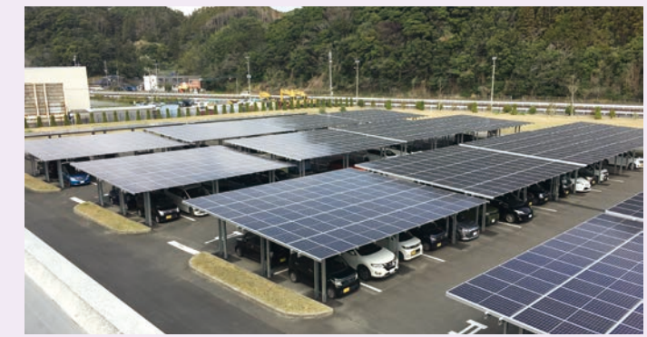
Solar panels at the entire parking area to produce electricity for internal use
