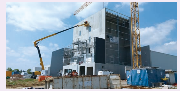
Construction of a spray dryer in France
