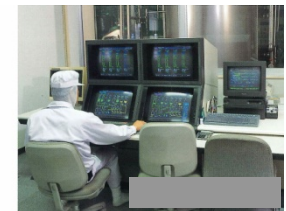
Computer control room
